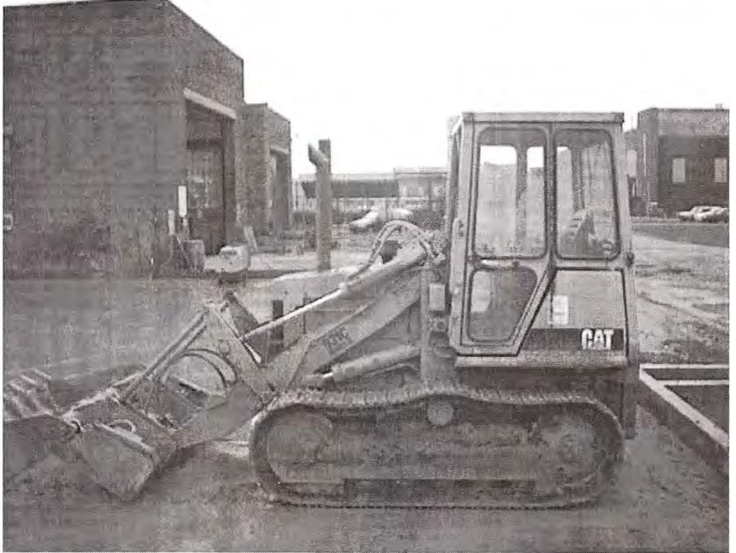
Tracked Loading Shovel
