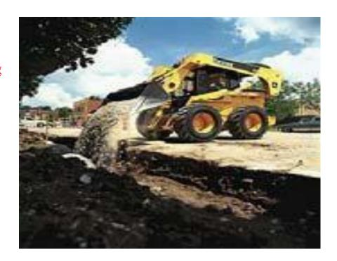
Always use stop blocks or earth beam banks when discharging materials into the trench
