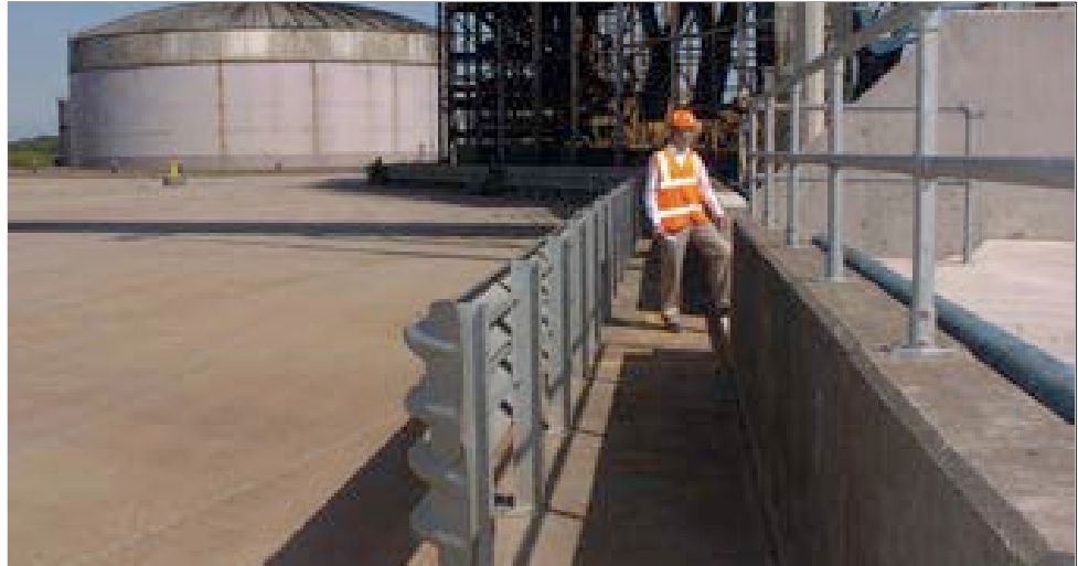
Figure 1 Barriers to protect pedestrians
