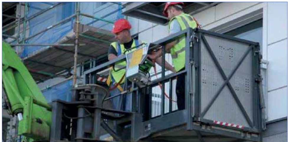
Figure 19 Integrated working platform
