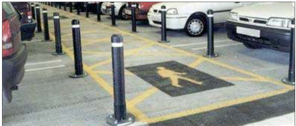
Figure 9 Pedestrian walkway in car park
