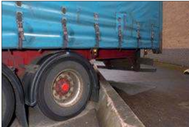
Figure 7 Concrete wheel stop
