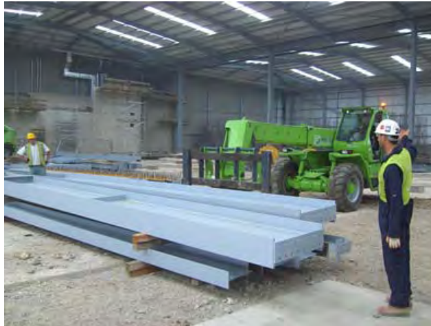
Figure 19 - Use of Wider Fork Carriage
